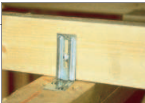
Shrinkage in bottom chords and expansion in top chords cause trusses to flex upward at the center, lifting walls and ceilings with them. Prevent the problem with truss clips (left), which allow the truss to move up and down with seasonal moisture changes, while restraining movement in any other direction.
