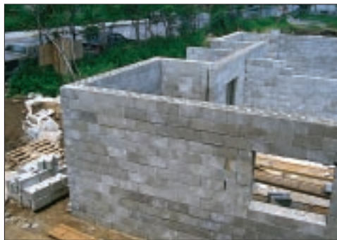
The Sparfil Wall System allows one-step construction of a fire-rated structural wall, complete with insulation and air barrier.
