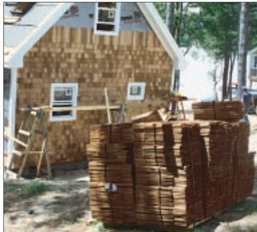
Cedar shingles are still plentiful, but quality varies from mill to mill, and grading has been inconsistent.
