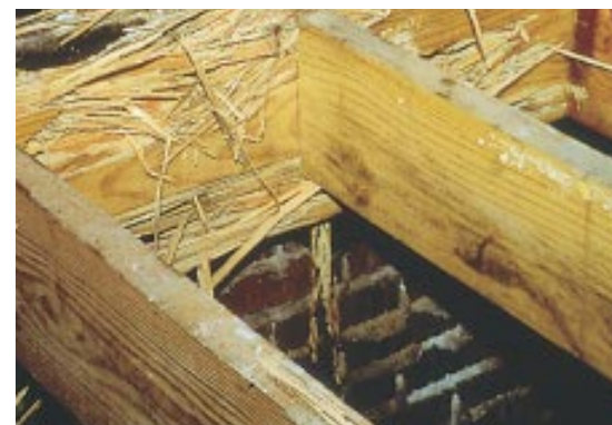
Formosan termites, imported accidentally from China, devour wood much more aggressively than native termite species. New Orleans, where this picture was taken, has been particularly hard hit by infestations.
