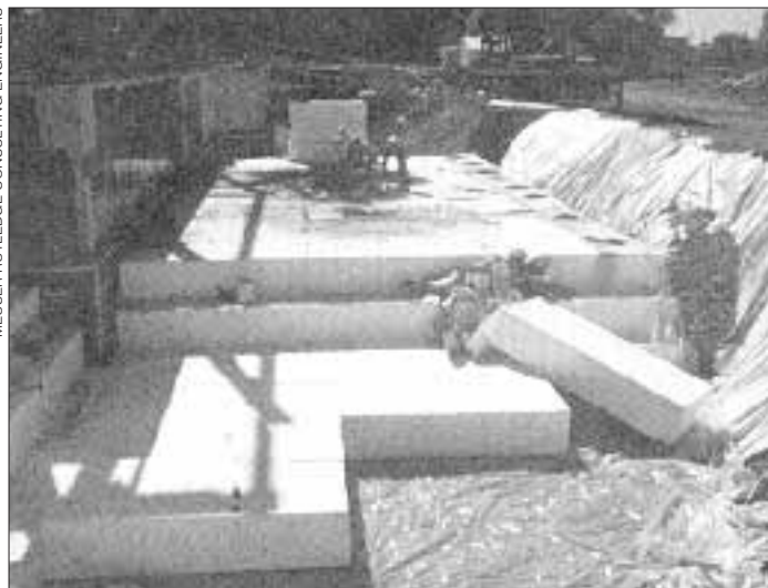
Large polystyrene blocks placed as lightweight backfill around this suburban Syracuse mall reduced the settling of the unstable soils and prevented foundation problems.
