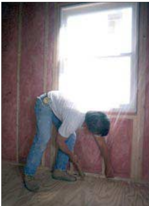
Clear plastic vapor barriers were first used in Canada to allow for easy inspection of insulation, Energy Design Update reports.
