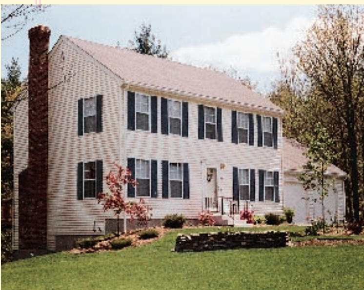
Simple floor plans and traditional designs are staples of Bovenzi Inc.'s homes, which range from multi-unit apartment complexes to traditional three-bedroom Colonials like this one.
