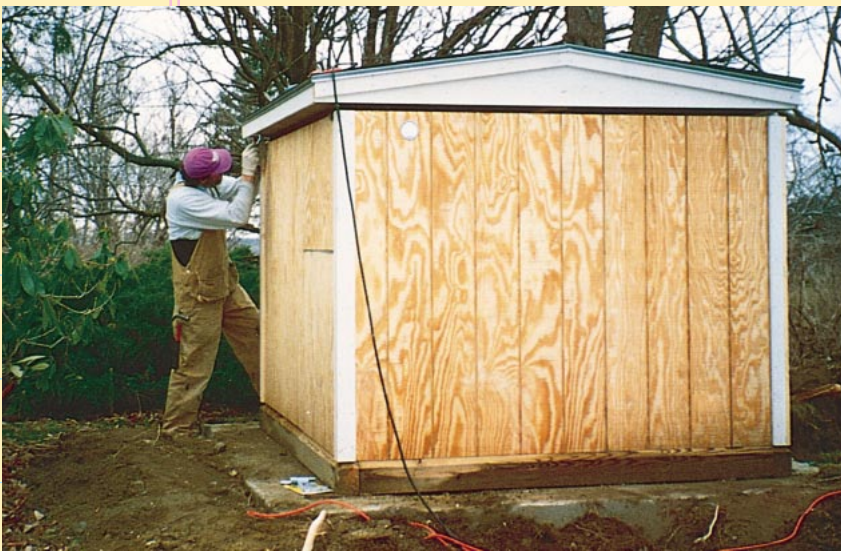
This small building houses a site-constructed “biofilter” for treating residential wastewater. The effluent from the septic tank is sprayed over a foam plastic medium, which cleans the waste water before it is pumped to a small leach field.
