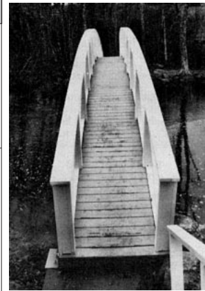
The handrail is a laminated 2x8, lag-bolted to the baluster caps. The diagonal supports are 4x4s, nailed into place.
