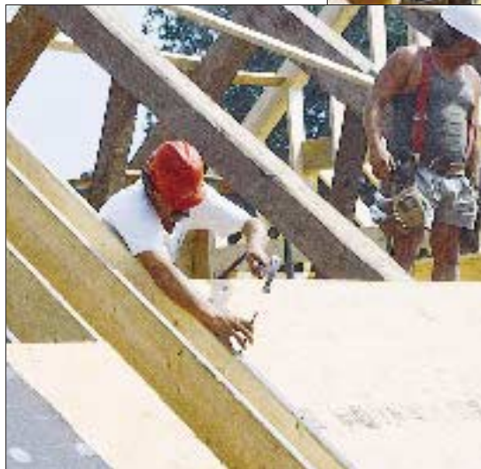
Stress-skin panels provided insulation, interior blueboard base for veneer plaster, and exterior sheathing.
