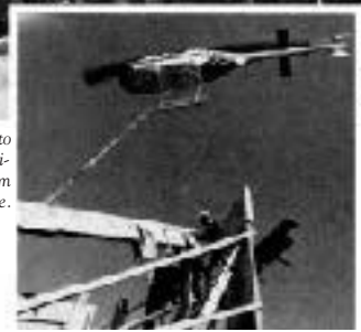
All of the 42-foot beams were airlifted to the island and set in place by the helicopter. While the helicopter held the beam (inset), the crew bolted it into place.
