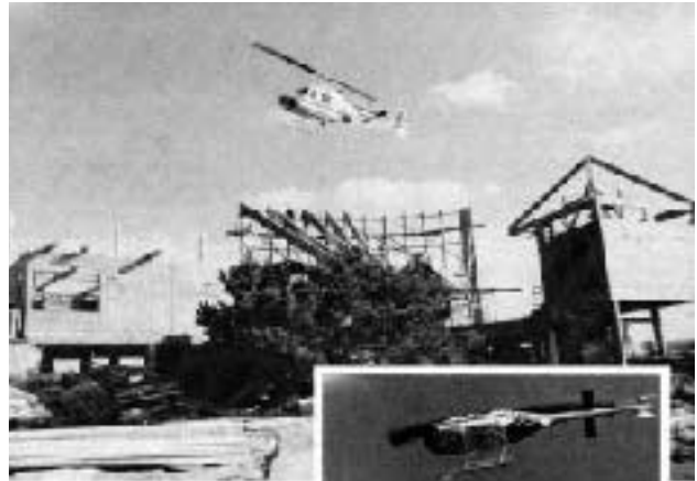
All of the 42-foot beams were airlifted to the island and set in place by the helicopter. While the helicopter held the beam (inset), the crew bolted it into place.
