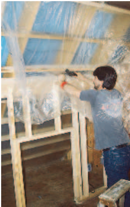
Figure 5. In the case shown, a kneewall complicated the vapor barrier installation (photo, left). To prevent that, the author recommends first insulating the entire roof plane down to the eaves, then building the kneewall. Besides giving a 13-inch-deep insulation cavity, the crisscross build-down also provides a 2 1 / 2 -inch thermal break below the rafters (illustration, right).
