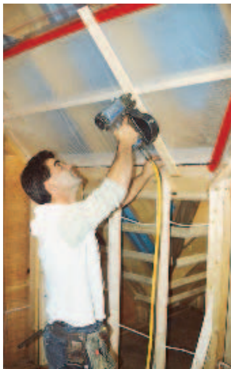
Figure 4. The author's newest method is to spike 2x3s on edge crosswise to the rafters (left), install a reinforced vapor barrier and strapping (center), then blow the cavities with cellulose (right).
