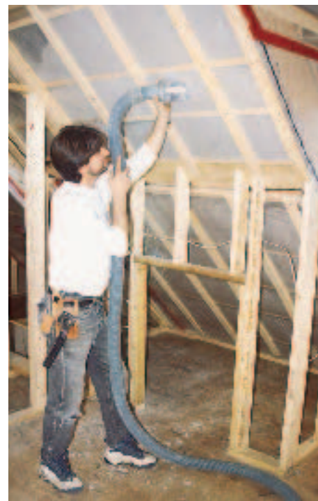
Figure 4. The author's newest method is to spike 2x3s on edge crosswise to the rafters (left), install a reinforced vapor barrier and strapping (center), then blow the cavities with cellulose (right).
