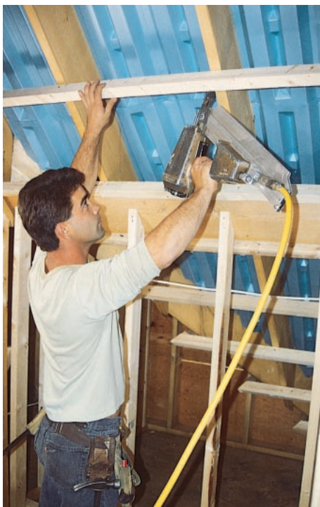
Figure 4. The author's newest method is to spike 2x3s on edge crosswise to the rafters (left), install a reinforced vapor barrier and strapping (center), then blow the cavities with cellulose (right).
