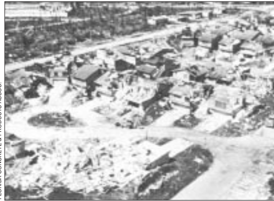
FLORIDA CONCRETE & PRODUCTS ASSOC.
