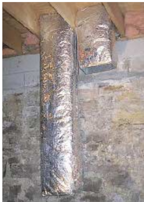
Figure 5. In this basement, which is too small to be considered an unconfined space, two ducts provide combustion makeup air from the exterior. One duct terminates near the ceiling, and the other terminates near the floor. The air intakes are protected at the exterior with rain hoods and screening.
