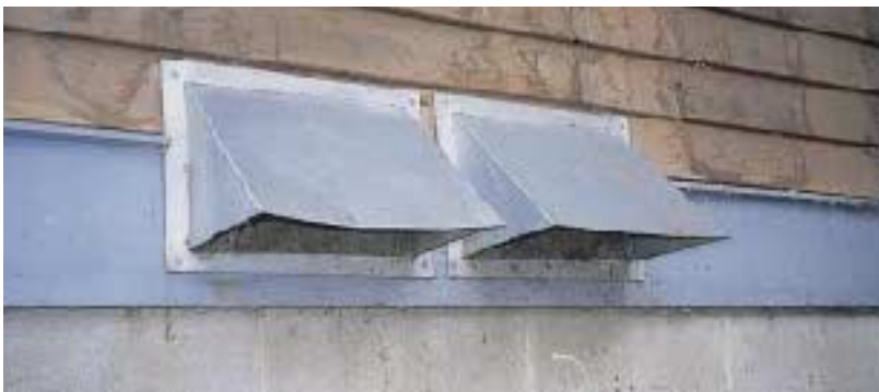
Figure 5. In this basement, which is too small to be considered an unconfined space, two ducts provide combustion makeup air from the exterior. One duct terminates near the ceiling, and the other terminates near the floor. The air intakes are protected at the exterior with rain hoods and screening.
