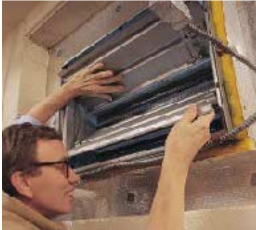
Figure 6. Motorized dampers are installed in very cold climates, where exterior makeup air might be cold enough to freeze plumbing pipes in a utility room or basement.
