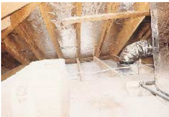
Figure 3. Foil radiant barriers can reduce unwanted heat gain by up to 40%. The foil barrier should be installed on the underside of the sheathing and should be cut at the ridge vent to allow heated air in the attic to escape.
