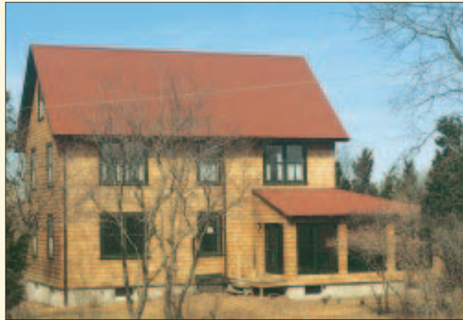
Figure 1. The author's project house looks fairly standard, but careful detailing makes it highly energy-efficient.
