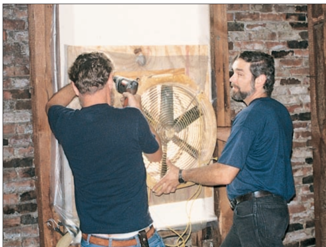
A worker preparing to spray-apply urethane masks a skylight (above) and hooks up an outside air supply to his respirator (above left). An exhaust fan (left) pulls hazardous fumes from the work area. The actual spray job takes only a few hours (below left).
