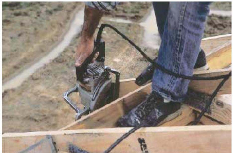
Figure 7. Truss tails are marked with a string (top) and cut plumb.
