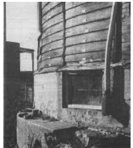
The first-floor plan (above left) features an oval living room, a round library with two alcoves, and an elegant elliptical stair. Floors and ceilings were framed radially (above right) like a spiderweb. Foundation parging colored to mimic brownstone (right) awaits repair, as do the tagged and catalogued pine clapboards.
