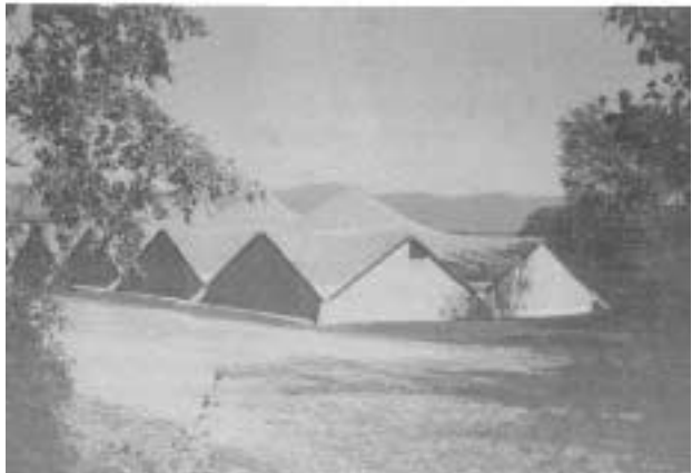
Hypars can join one to the next to form a graceful roofscape, such as on this field house at Vermont's Middlebury College.
