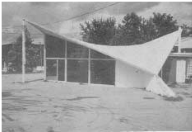
A gas station roof makes good use of the saddle-shaped hypar.
