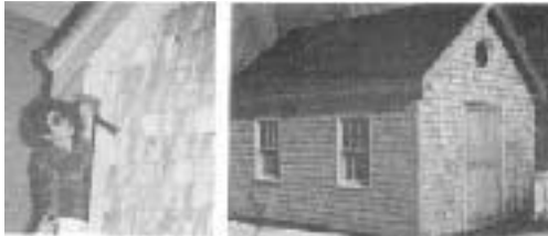
A 12x16-inch multi-purpose building (right) was constructed last Fall by a class at The Women's Trade Center (WTC). It took one month to complete. The building was sold to be used as a summer camp in Warren, Maine, and has no heating, wiring, or plumbing. WTC's director Cathy Stiles is shown finishing up (left).
