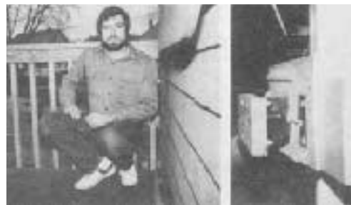
General contractor Rick Jewell shows how the deck bracket he used on a deck in Auburn, Maine, can provide a breathing space between the deck and the main structure, preventing deterioration from trapped moisture. The bracket can be seen more clearly in the demonstration model shown at right.
