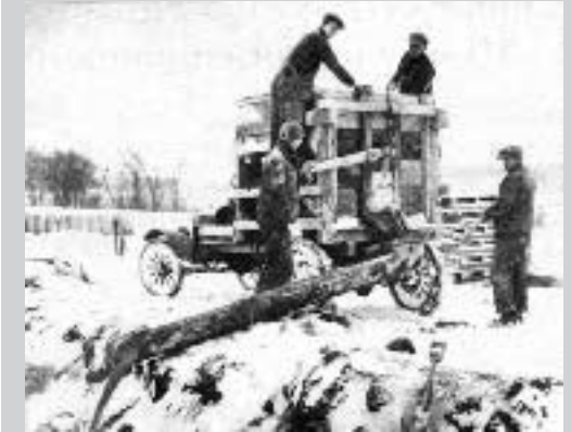
Ready-Mix Prototype: This first-generation cement mixer is delivering fresh concrete to pour the foundations for the Ford Plant in St. Paul, Minn., circa 1919. Photo courtesy of Schewing America, Inc (White Bear, Minn.)
