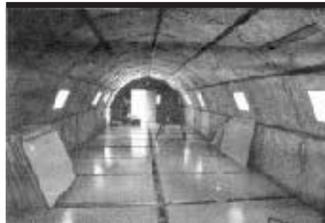
Finished modulares are 45 feet long; interior space is 15-foot wide, with 9-foot 4-inch vaulted ceilings.
