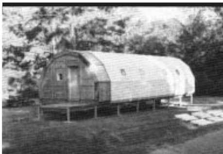
Modular-plastic cladding attaches rapidly without fasteners, interlocking to form a weatherproof shell.
