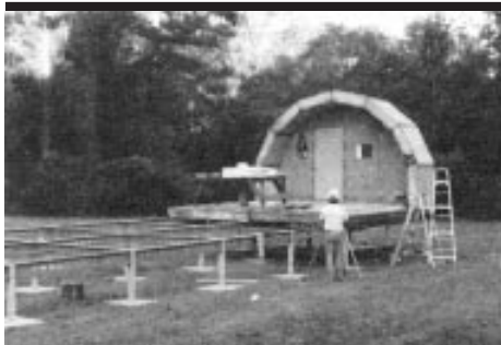
Assembly of Hypertat units requires no special skill or tools and can take less than 8 hours for two people.
