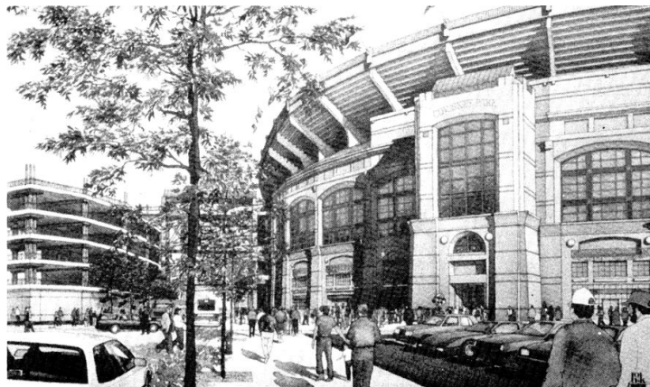
The design of two baseball stadiums, one in Chicago and one in Baltimore, will mimic the design of stadiums built at the turn of the century. Chicago's Comiskey II (illustrated above) will even use precast concrete to mimic the brick facade of aging Comiskey park.
