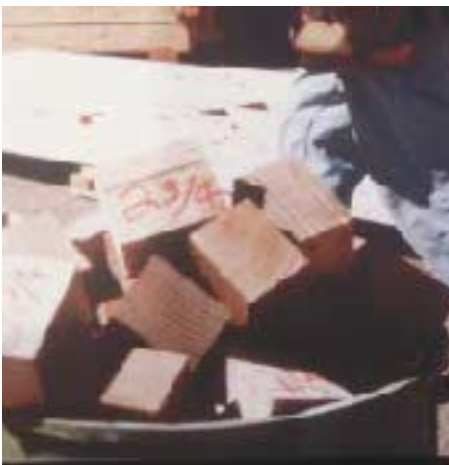
Figure 5. These timber cutoffs have been salvaged from the scrap pile and ripped down to 2 3 / 4 inches for use as cripples. This eliminates splitting problems, reduces waste, expedites assembly, and improves quality.
