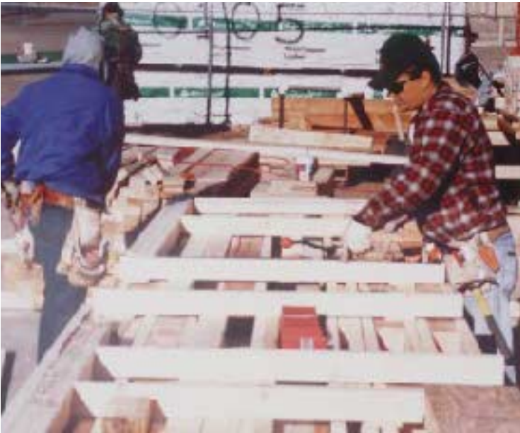
Figure 1. Everything is fitted carefully to keep freight costs down and create a tight, solid, stackable package that will help reduce warping (left). “Hybrid-prefab” packages contain everything you need to build walls, including pre-cut plates, headers, trimmers, channels, corners, nails, hardware, and drawings (right).
