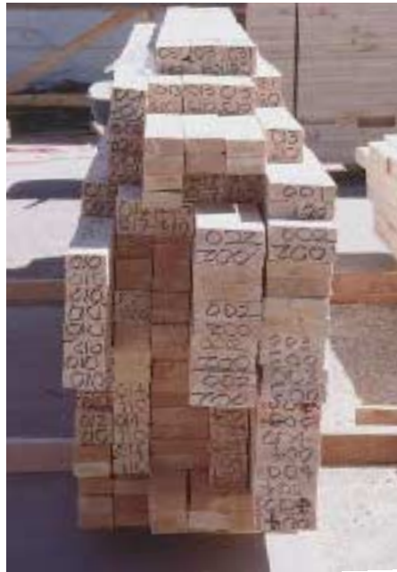
Figure 3. As wall plates are cut to length, they are labeled and nailed into sets (left). Pre-cut plates are then moved to the layout station, where stud and component placement, top plate length and positioning, anchor bolts, and “courtesy cuts” at doorways are laid out (right).
