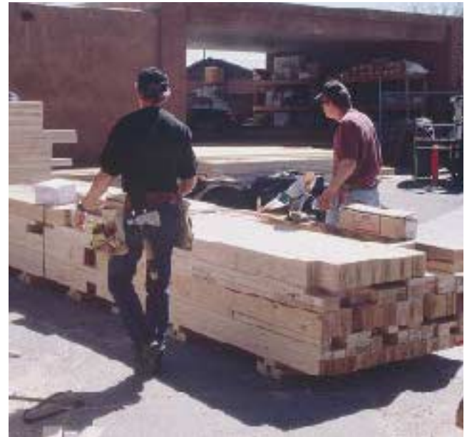
Figure 1. Everything is fitted carefully to keep freight costs down and create a tight, solid, stackable package that will help reduce warping (left). “Hybrid-prefab” packages contain everything you need to build walls, including pre-cut plates, headers, trimmers, channels, corners, nails, hardware, and drawings (right).
