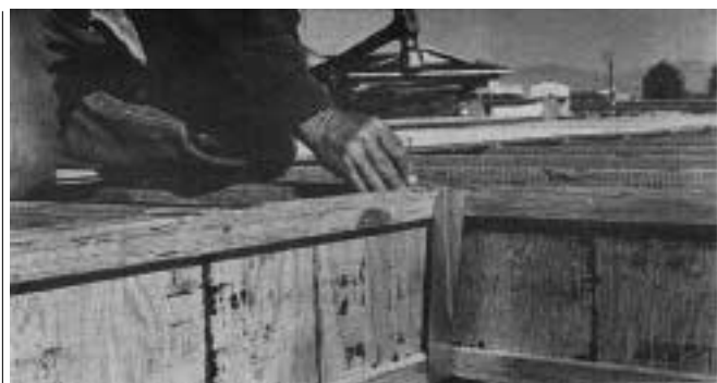
Plywood I-beams from Trus Joist use 2x wood chords and webs of vertical-grain plywood. Primary uses: floor joists and rafters.
