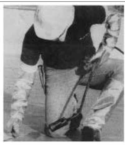
Modified bitumen (above) is essentially built-up roofing on a roll, but is easier to seal at penetrations and flashings. One type is sealed with hot asphalt, another uses a torch (left).
