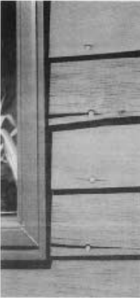
Splitting (above) and nail popping (right) are common on horizontal wood sidings installed directly over foam sheathing. One solution is to put the foam on the inside.
