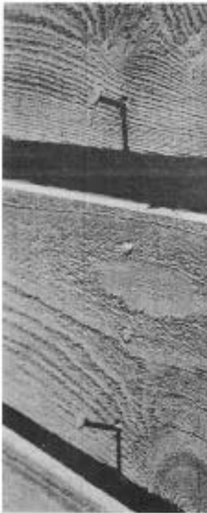
Splitting (above) and nail popping (right) are common on horizontal wood sidings installed directly over foam sheathing. One solution is to put the foam on the inside.
