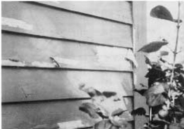
No primer here led to poor adhesion and wholesale peeling to bare wood. One telltale sign was no trace of any white pigment on the wood or the back of the paint chips.
