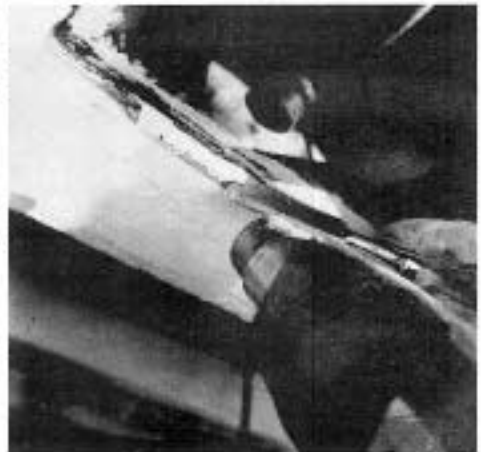
Use a heat gun on stubborn spots, then scrape the putty out with a chisel. This is risky for glass you want to keep. You can use a putty knife as a heat shield. Alternate tool: 2- or 3-lb. soldering iron.
