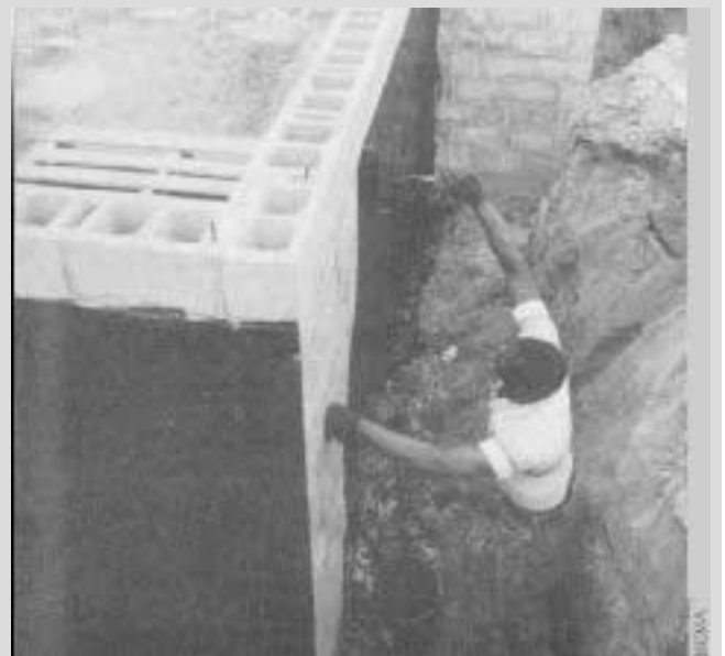
Damp-proofing is not waterproofing. It blocks the flow of water vapor and water under slight pressure. But it won't hold off water under sustained pressure.
