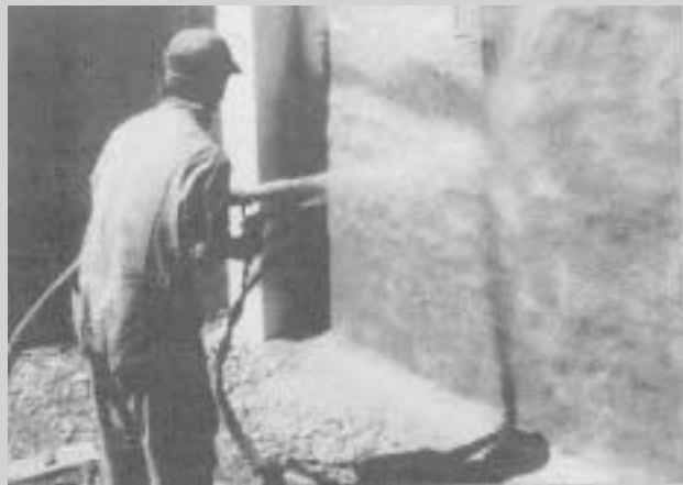
True waterproofing requires a continuous barrier against water. This system uses spray-on bentonite (Bentonize), a clay that expands when wet sealing off all leaks.
