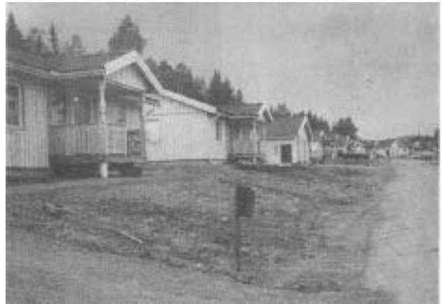
Scan-American will set up a temporary plant anywhere in the U.S. where it has negotiated contracts for 200 houses or more. Scan-American house components were used to build this single-family development in Colorado.
