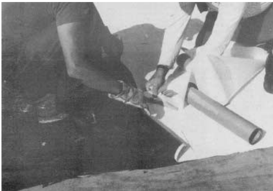
Just peel off the release paper and stick down the membrane. This ease of installation makes self-adhering bitumen roofing very attractive to residential contractors.
