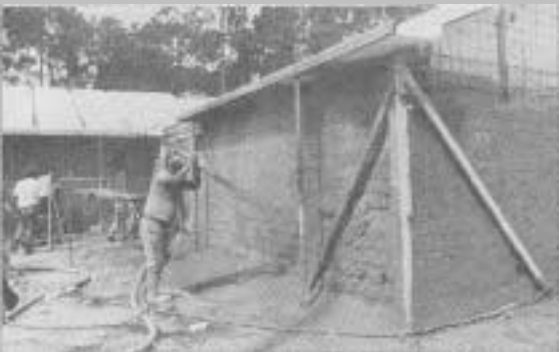
Shotcrete applied on exterior 2 inches thick.
