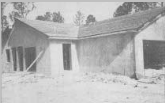
Completed wall ready for cladding.
