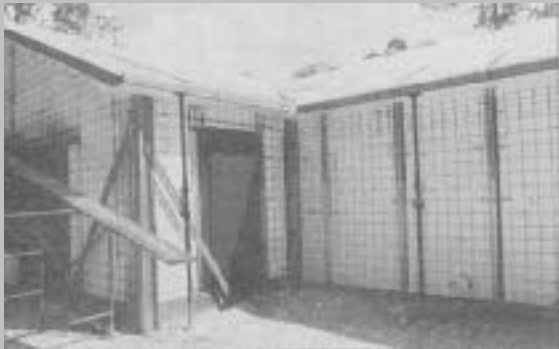
Polystyrene, wire mesh, reinforcing steel ready for shotcrete.
