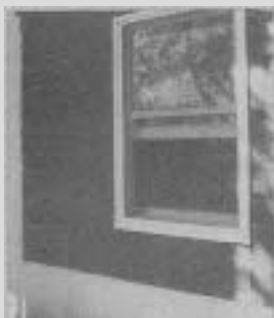
Downsizing an opening to fit stock windows saves both in replacement costs and energy use.
