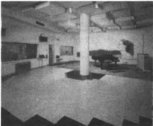
A sand-filled concrete-block wall goes up just inside the existing wall of the warehouse (top). The completed studio (bottom) has an array of boxes on the ceiling to diffuse sound. The large mural on the far wall disguises one of several sound-absorber panels made of Owens Corning Type 703 rigid fiberglass.
