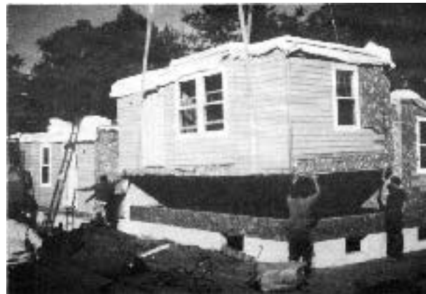
Some manufacturers may require that the builder obtain and pay for the crane used in installation.
