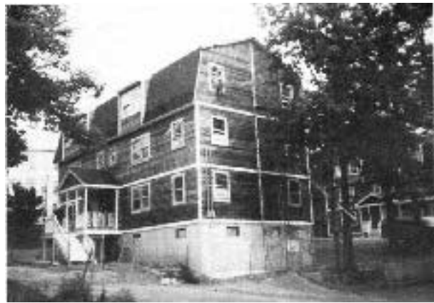
Virtually any kind of structure can be built with modular housing.
