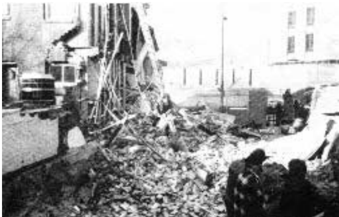
This masonry building collapsed when vibrations from heavy machinery caused the footings to slip into an excavated area.
