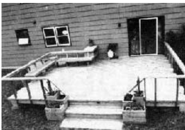
Figure 1. Offsetting the doorway to one side keeps traffic flow out of functional areas. Also, note how the decking patterns define different areas.
