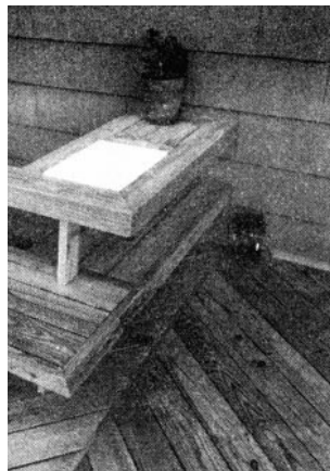
Figure 10. An inlaid section of Corian acts as a food counter and keeps food from contact with pressure-treated lumber.
