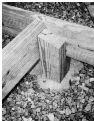
Figure 5. When setting posts, put the factory end down. Cut any exposed post tops at an angle to shed water, and always seal your cuts with a preservative.
