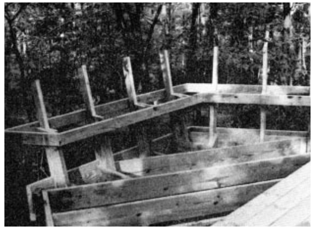
Figure 11. Notched 2x8s provide support for both bench seats and backs.
