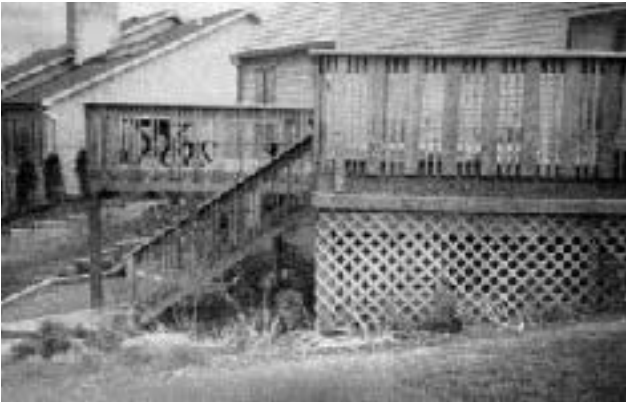
Figure 9. Different railing styles can define and separate functional areas on the deck. For sturdiness, screw rather than nail the railings. This also prevents splitting.
