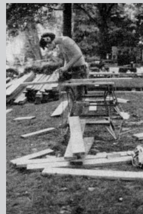
The cautious approach: The EPA recommends wearing a mask when sawing pressure-treated wood, and washing your hands before eating or smoking.
