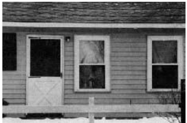
Figure 2. Vinyl (PVC) windows replaced single-pane aluminum windows in this tract home. In cold climates, this thermal upgrade makes sense.
