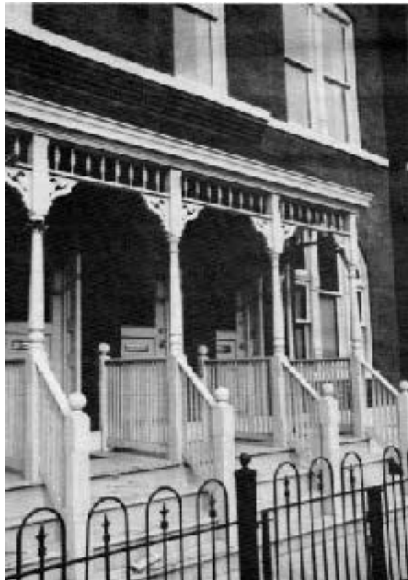
Figure 4. Stock parts from millwork companies create an instant vintage feel, but this new row house is actually high density—four units packed beneath the unifying porch.
