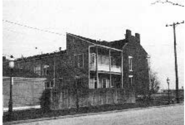
Figure 3. Brick fronts and sidewalls disguise this new construction. But the back of the building tells that it's infill—by the extended porch, balconies, integrated landscaping, greenhouse windows, and detached garages.
