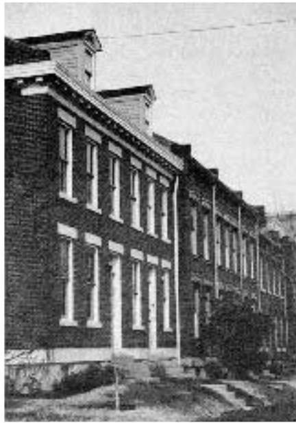
Figure 1. Built around a circular landscaped court, these townhouses (left) in St. Louis use stock parts to simulate a Victorian motif. Also in St. Louis, replica housing (right) looks like blocks of row housing. Cornices use fiberglass or brick dentils.
