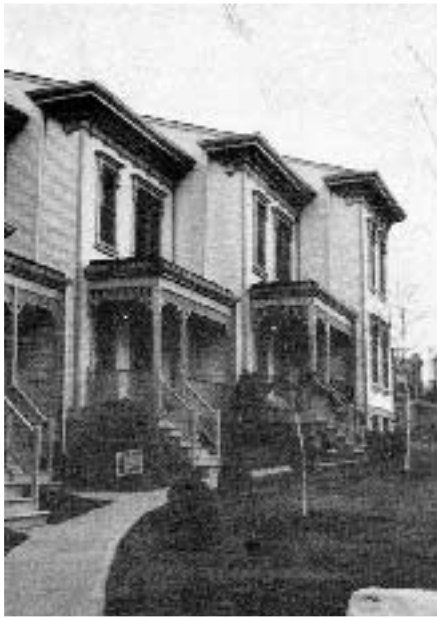
Figure 1. Built around a circular landscaped court, these townhouses (left) in St. Louis use stock parts to simulate a Victorian motif. Also in St. Louis, replica housing (right) looks like blocks of row housing. Cornices use fiberglass or brick dentils.
