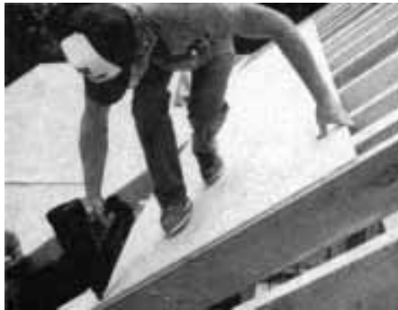
The Impulse nailer is powered by a small fuel cell and battery that frees the user from restrictive hoses and compressor. This can make roof framing and sheathing both faster and safer.
