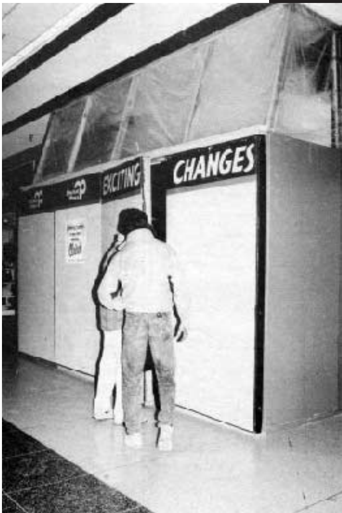
Mall managers want stores to remodel every five to six years. The contractor doing the job has to screen the job site and stay invisible.
