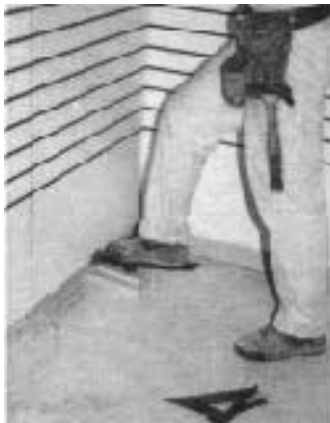
Figure 2. The author uses a drywall's foot lever (left) to position slat-wall panels in mitered corners. A screwgun (right) secures them in place. Shelves lock in the grooves.
