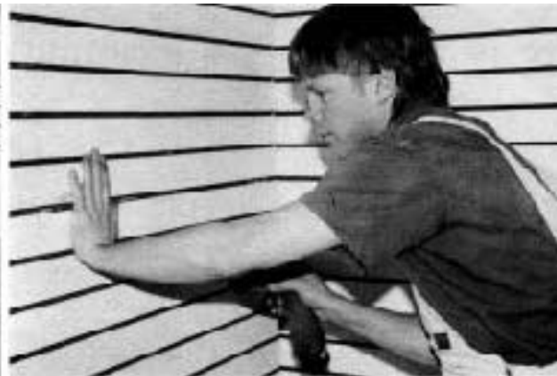
Figure 2. The author uses a drywall's foot lever (left) to position slat-wall panels in mitered corners. A screwgun (right) secures them in place. Shelves lock in the grooves.
