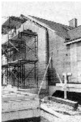
Figure 4. A free-standing masonry wall provides a 2-hour fire rating and excellent sound protection. One-inch spaces on either side of the wall leave the townhouse units structurally independent. The wall can be put up either before (above) or after (left) the adjacent units are framed.
