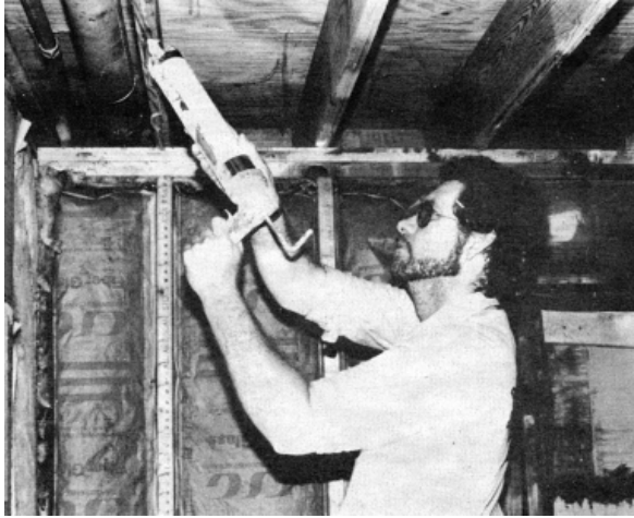
Figure 1. Panel adhesives reduce the number of nails needed to hang drywall. With some, you only need to nail the top and bottom plates.
