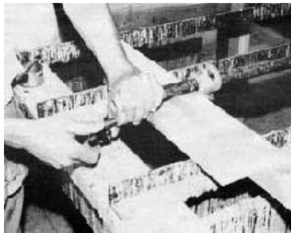
Figure 2. Yellow glue, used to glue cabinets, furniture, and other "frame" assemblies, must be clamped or held under pressure until the bond forms.
