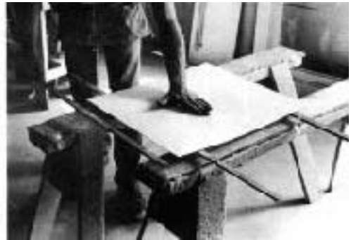
Figure 4. When working with contact cement, spray on two or three coats to seal the substrate if porous (left). Then position the laminate above spacers. Remove the spacers, (right) working from the center out, and roll or press thoroughly to form a bond.
