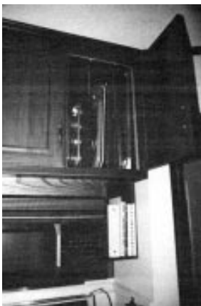
Figure 1. Minor on-site cabinetwork, such as this microwave surround, can dress up a refacing job. But with too much custom work, refacing is no longer a bargain.
