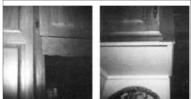
Figure 3. This new valance, at left, is locked in place with a narrow hardwood strip used to trim out the cabinet corner. The strip, at right, can also be set flush with the 1/4-inch veneer panel on the side of the cabinet.
