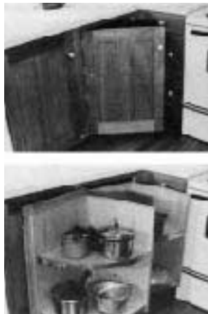
Figure 1. Two swinging "quadrant" shelves make use of the space in a corner base cabinet. One shelf is screwed onto the back of the door (note the four hinges at left, in top photo, needed to support it). The other is attached with a piano hinge to the inner edge of the cabinet's face frame.
