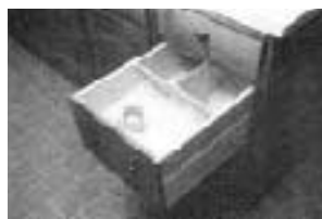
Figure 2. Drawers designed for heavy food items should extend the full length of the cabinet; the extra length is needed to counterbalance the added weight when the drawer is open. A sheet of copper, screwed to the back of the face-frame rail above the drawer, acts as a protective lid.
