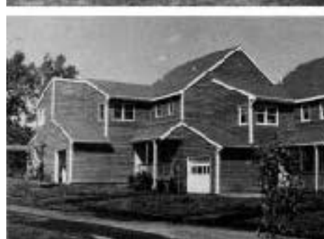
Figure 4. Building consultant Steven Winter helped builders design and develop these upscale townhouses in the N.Y. suburbs using the modular approach. Winter contends that almost any design can be built in modules.
