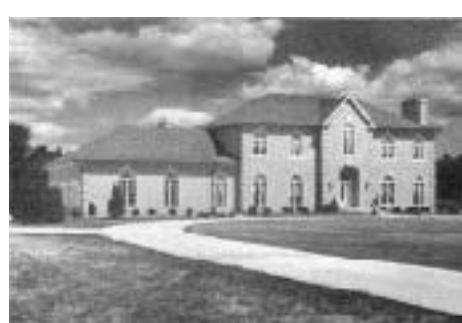
Figure 3. Modular producers like Nanticoke want nothing to do with the low-end "cookie-cutter" approach as the 4,000 square-foot house above demonstrates. This Delaware home was manufactured and shipped in four modules.
