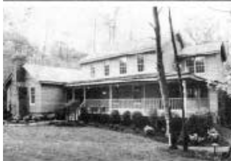
Figure 2. This 2,700 square-foot modular was built in Ryland's Fredericksburg, Va., plant based on a popular stick-built floorplan. Cedar siding and shakes, (top) were installed on site, while interior frills (bottom) arrived complete.
