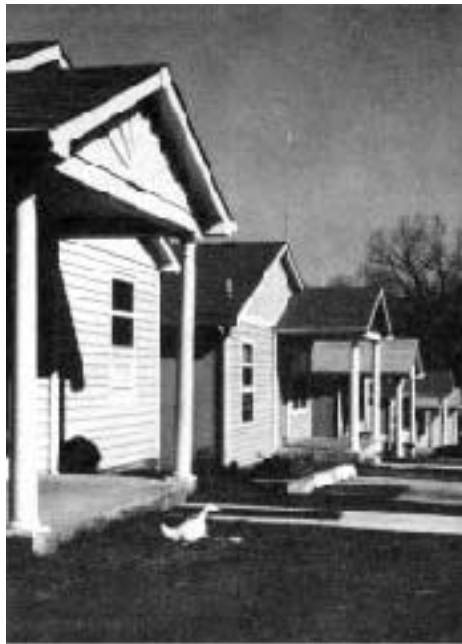
Figure 1. These 1,000-square-foot infill units were built for about $40 a square foot in Kansas City, Mo. Older urban neighborhoods are a growing market for lower-end modular housing.
