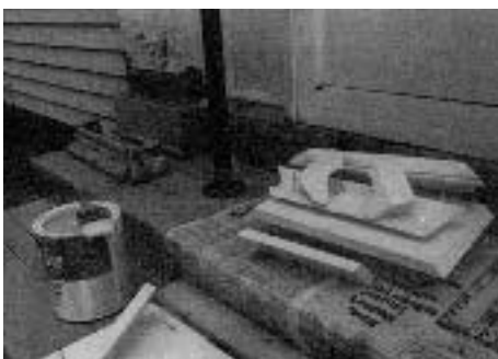
Figure 3. Pre-cut pieces of trim, with nails in place, await priming. The nails provide a handy way to hold the trim when priming.
