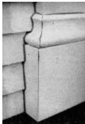
Figure 4. The author applies caulk to the mating faces of trim before installation. Excess caulk that squeezes out is cut or sanded away. An additional 1/8-inch bead of caulk finishes the joint between clapboard and pilaster.
