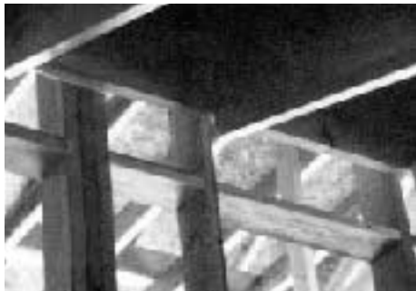
Figure 2. Where a cathedral ceiling meets an exterior wall that extends up past the ceiling, use blocking in the wall to prevent infiltration of moist household air into the ceiling cavity.
