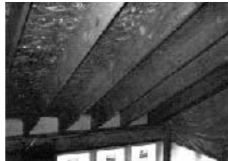
Figure 3. Foam blocks at the bottom of a rafter-framed cathedral ceiling will prevent cold air intrusion into the insulation near the eaves. The blocks should be caulked in place to ensure a good seal.
