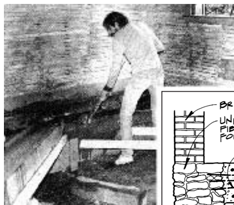
Figure 4. The grade beam was poured on all sides of the perimeter of the building. Rebar tied it to the ground and the fieldstone foundation wall.
